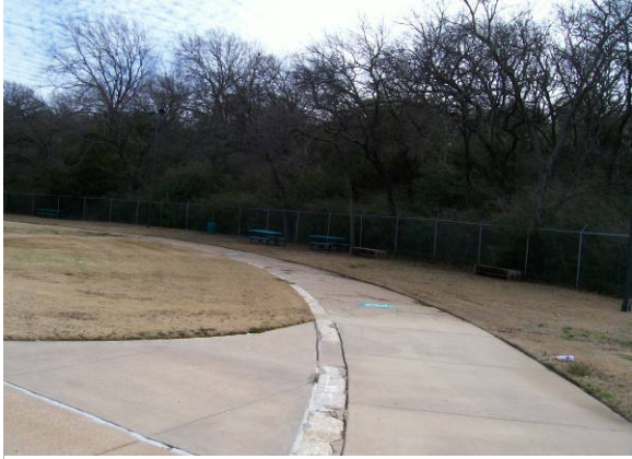
Original 1922 pool shell is deteriorating.
