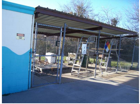
Covered mechanical space and adjoining chemical room.
