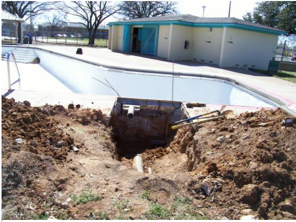
Equalizer tank replacement in progress
