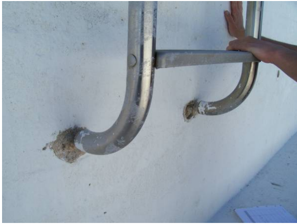
Without the rubber feet this ladder is wearing holes into the pool shell. (Reported to be repaired during annual maintenance for 2007 season.)
