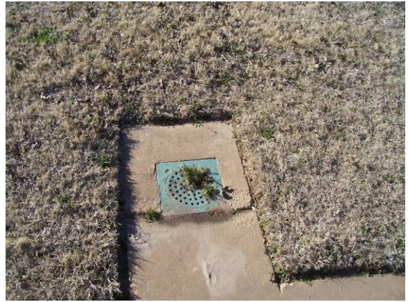
Area drains are filled with soil and vegetation. (Reported to be repaired during annual maintenance for 2007 season.)
