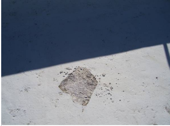
Rough pool shell surface
