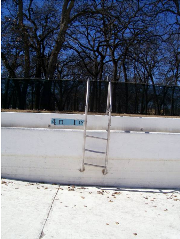
Ladders are in poor condition. (Reported to be repaired during annual maintenance for 2007 season.)
