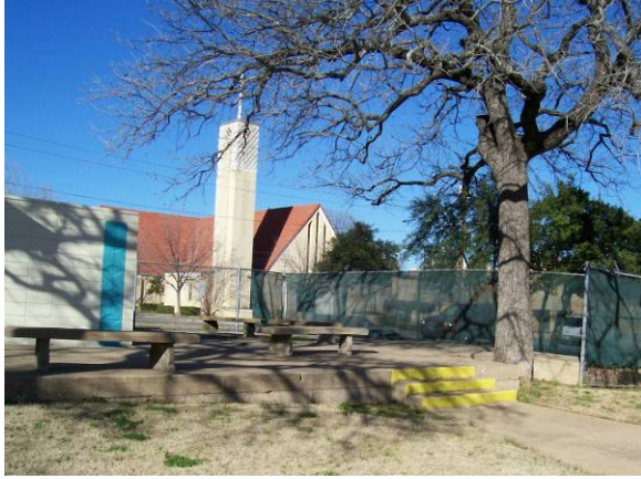
Hand rails not provided for stairs. Safety barrier not provided along front edge of patio.
